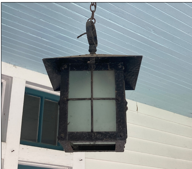
Character defining light fixtures must be retained. Photograph by Loggia Preservation, 2025.
