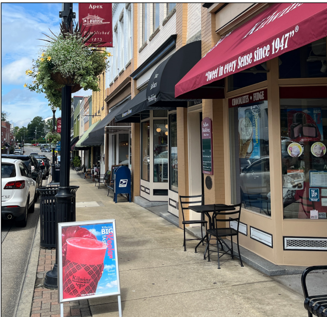
Signs must be appropriately scaled to the historic building and located to avoid obscuring or damaging historic materials. Photograph by Loggia Preservation, 2025.
