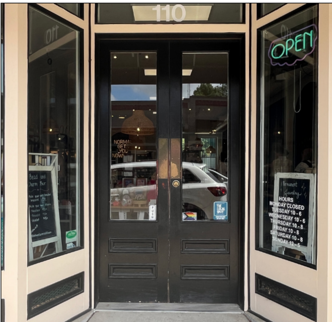
The paired wood doors are the centerpiece of the storefront entrance of the Sellars Building in Apex. Photograph by Loggia Preservation, 2025.
