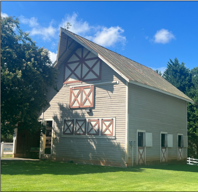
This accessory structure is a contributing outbuilding associated with the Wakefield Barn, near Wake Forest, and reflects the property's historic use as a dairy farm. Photograph by Loggia Preservation, 2025.
