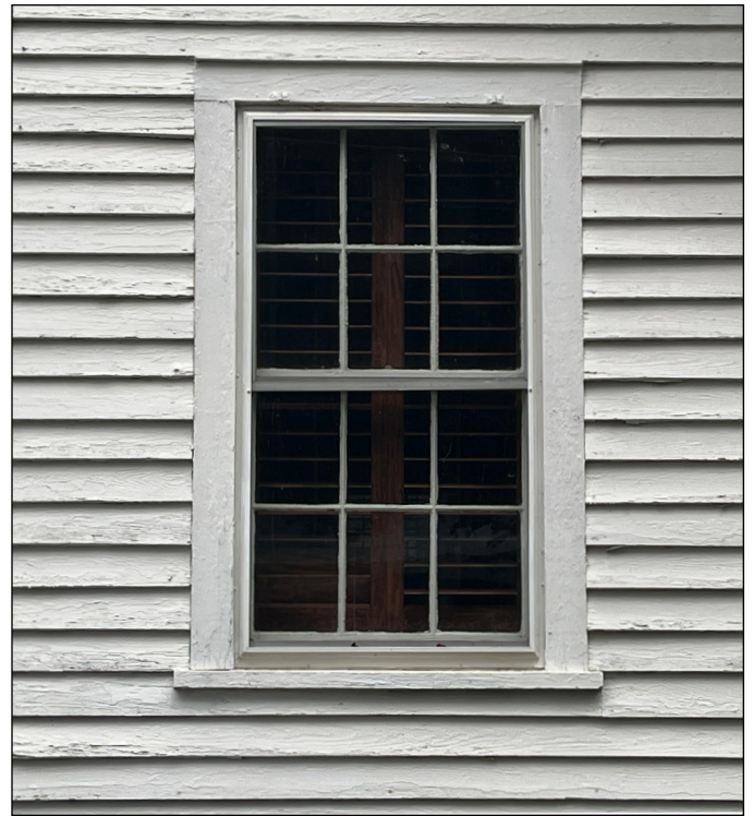
Storm windows must be installed so that the historic sash and detailing remain fully visible, as illustrated at the Fuquay-Varina Women's Club building. Photograph by Loggia Preservation, 2025.
