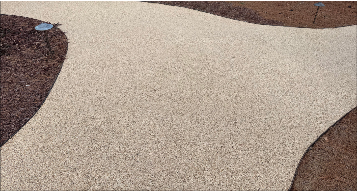
A stabilized aggregate walkway provides the appearance of a natural gravel path while creating a durable walking surface. Photograph by Capital Area Preservation, Inc.
