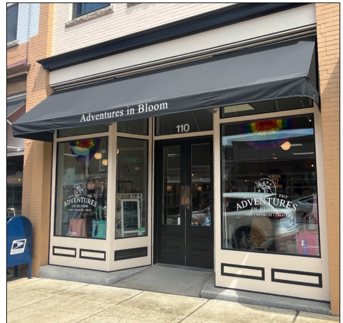
Lettering style, graphics, and finishes must be historically compatible. Photograph by Loggia Preservation, 2025.
