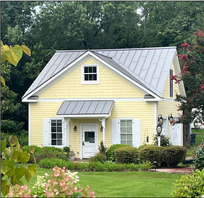
A contemporary outbuilding compatible in scale, form, and materials is sited to remain secondary to the historic residence at the Harward House in Apex. Photograph by Loggia Preservation, 2025.
