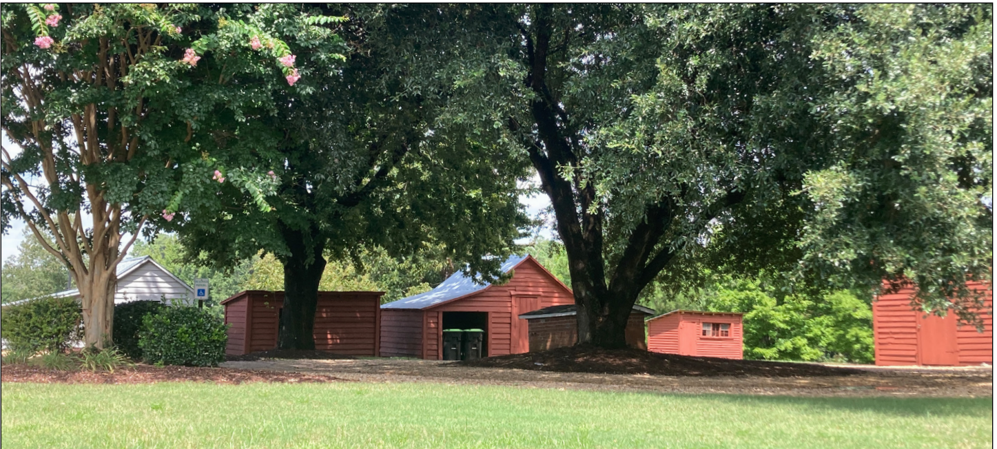
Outbuildings such as barns, milking sheds, and chicken coops are essential components of many historic landmark properties. Photograph by Loggia Preservation, 2025.
