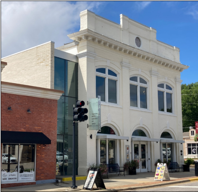
A contemporary addition to the former Apex Town Hall is differentiated from the historic building while maintaining compatible scale and form. Photograph by Loggia Preservation, 2025.
