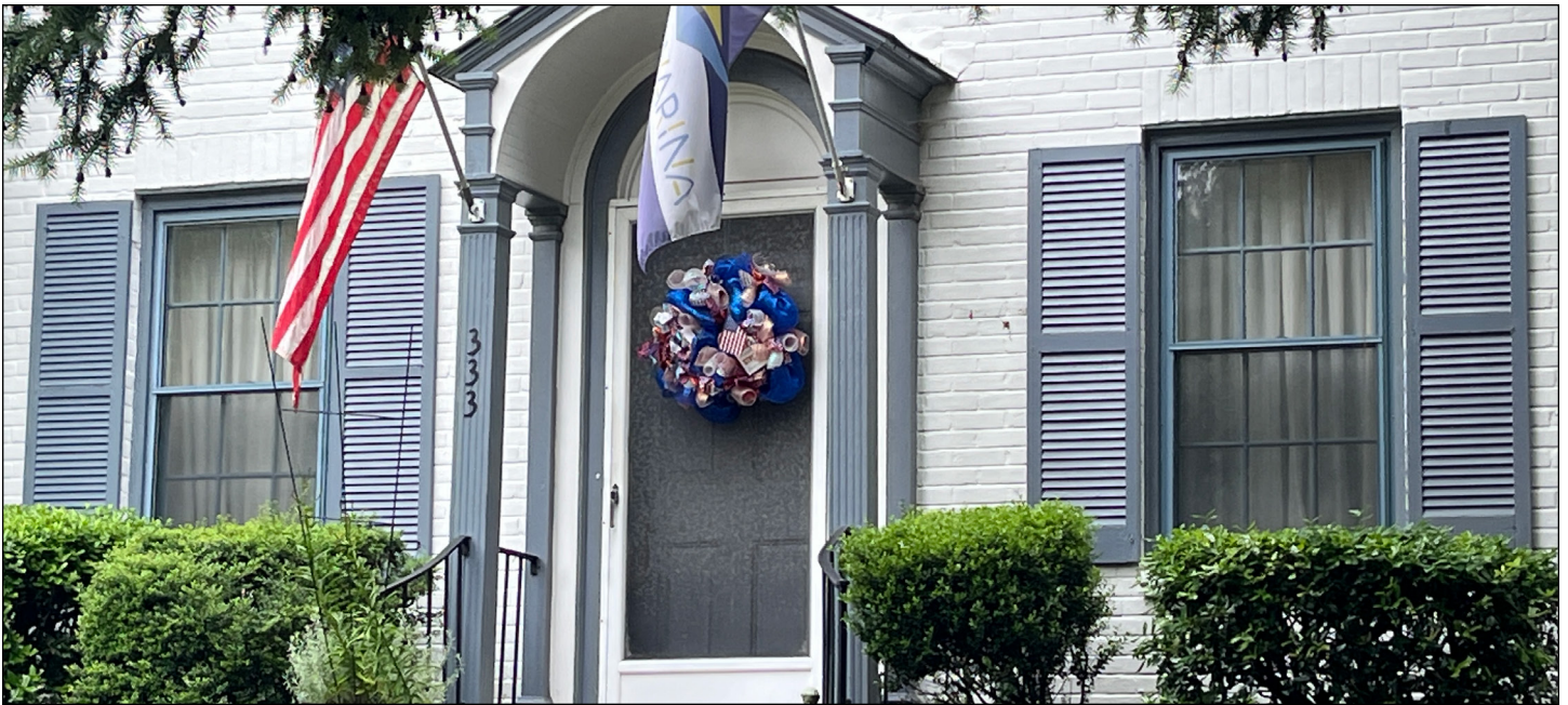
Storm windows must match the color of the existing sash and align with the muntin divisions, as shown above on the Dr. Wiley S. Cozart House in Fuquay-Varina. Photograph by Loggia Preservation, 2025.
