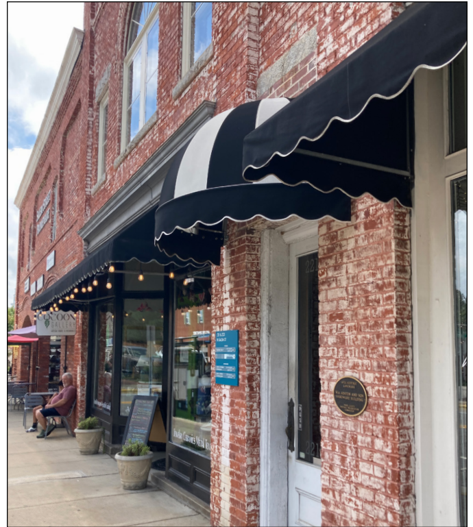
Sloped fabric awnings above storefront openings at the Hinton and Son Hardware Store in Apex. Photograph by Loggia Preservation, 2025.
