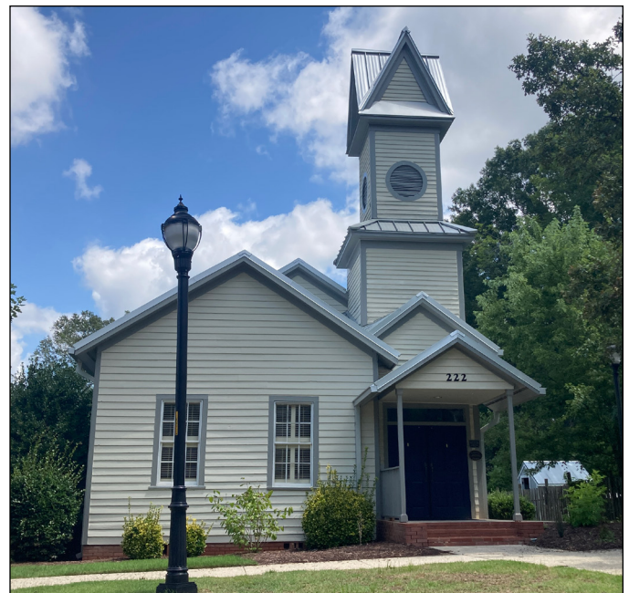
Contrasting paint defines the window surrounds, rooflines, and trim of the Morrisville Christian Church. Photograph by Loggia Preservation, 2025.
