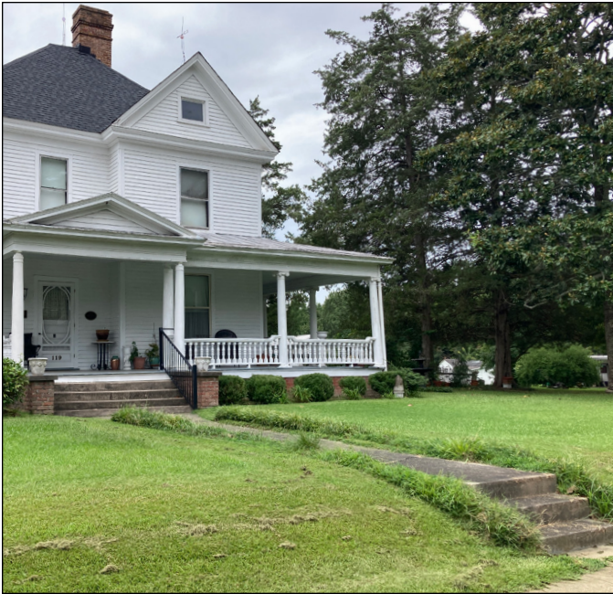
Historic site grading, slopes, and topography were often intentionally designed to manage drainage and protect the building from water as shown at the Dr. Lawrence Branch Young House in Rolesville. Photograph by Loggia Preservation, 2025
