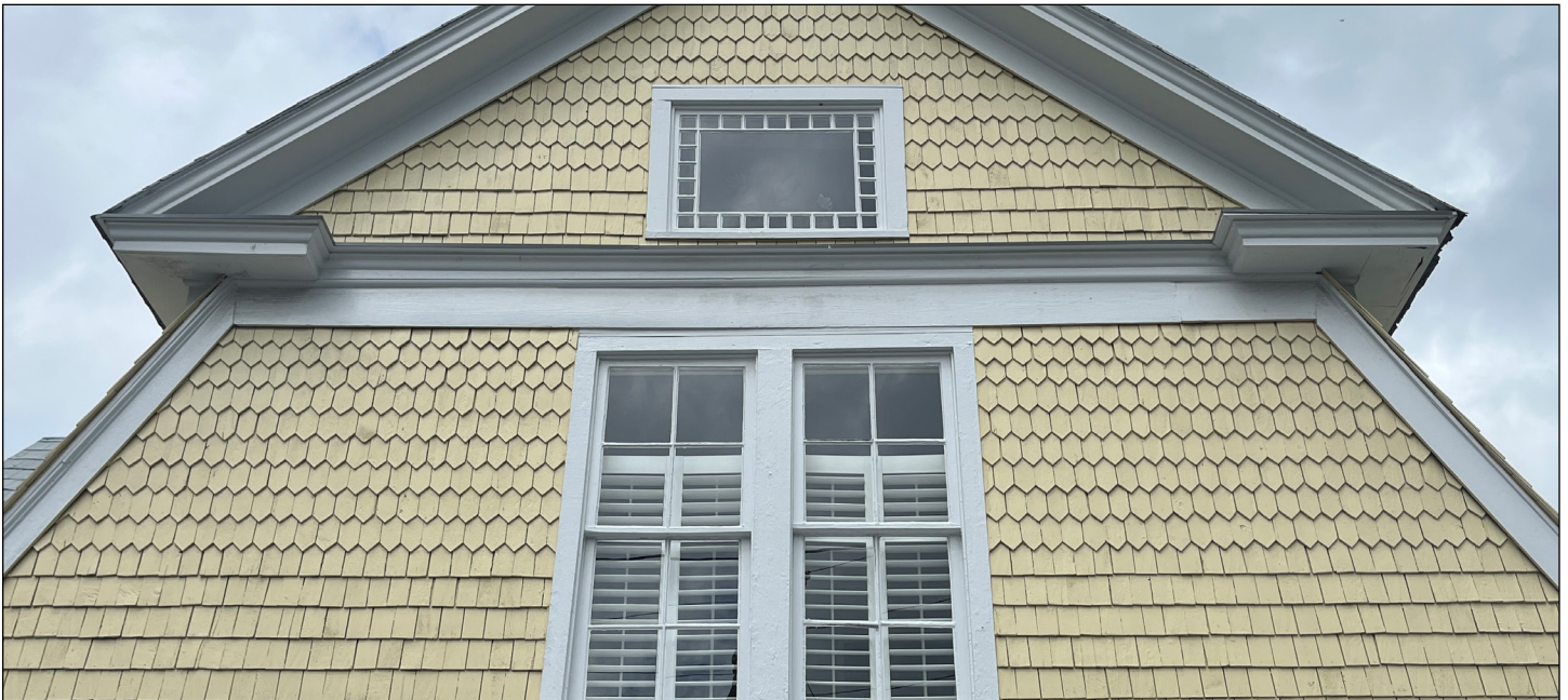
The wood shingles and trim are character-defining features of the Queen Anne-style Harward House in Apex. Photograph by Loggia Preservation, 2025.
