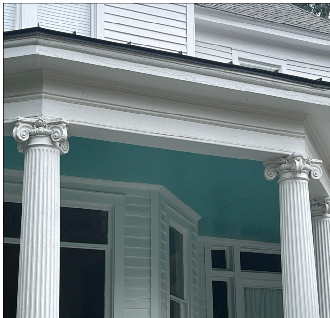
Fluted columns, decorative capitals, entablature, and painted porch ceilings are character-defining features at the Walter-Aiken House in Fuquay-Varina. Photograph by Loggia Preservation, 2025.
