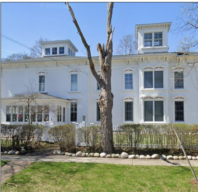
Additions that imitate the original architectural style, like the addition on the right shown here, create a false sense of history and are not appropriate. Photograph from Google.
