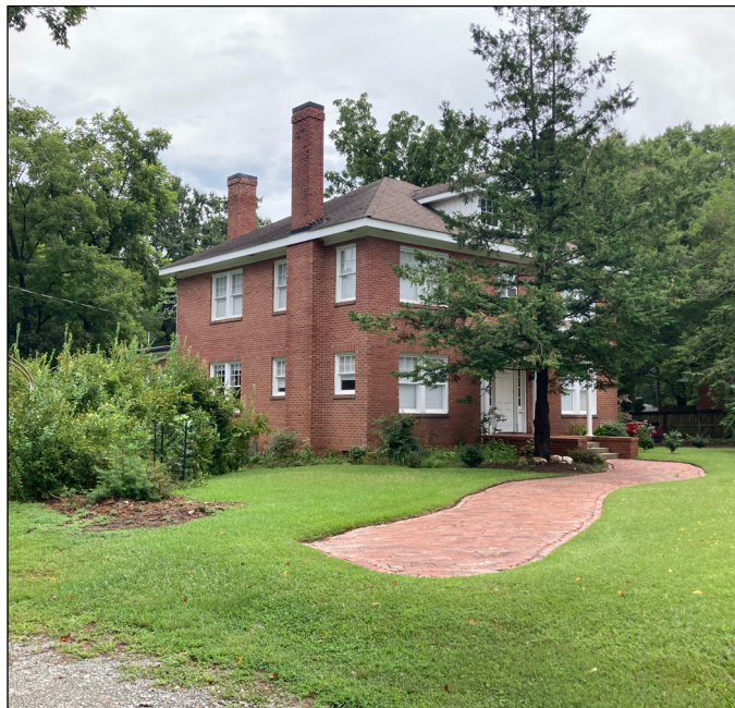
Hardscaping must follow existing topography and avoid unnecessary grading or landform alteration. Photograph by Loggia Preservation, 2025.
