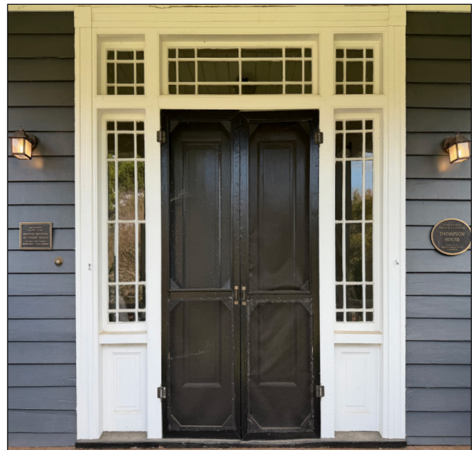
The primary entrance of the Thompson House near Wake Forest features an ornate door surround with a decorative transom and sidelights. Photograph by Capital Area Preservation, Inc.
