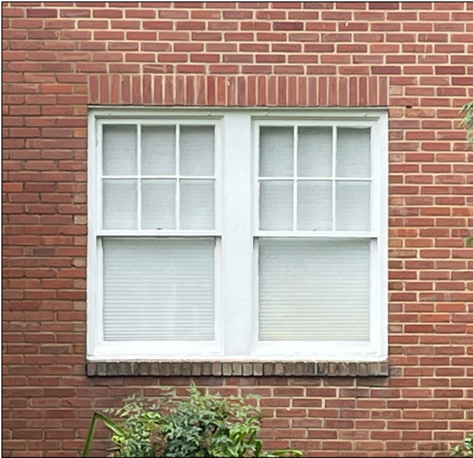
6-over-1 wood windows at the Wayland H. and Mamie Burt Stevens House in Fuquay-Varina are distinctive elements of the building's Colonial Revival exterior. Photograph by Loggia Preservation, 2025.
