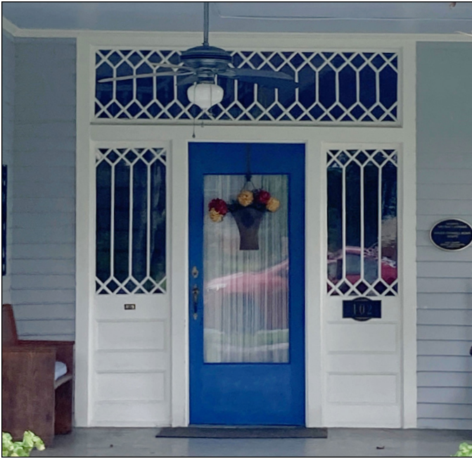
The primary entrance of the Hales-Tunnell-Bunn House in Wendell features an ornate door surround with a decorative transom and sidelights. Photograph by Loggia Preservation, 2025.
