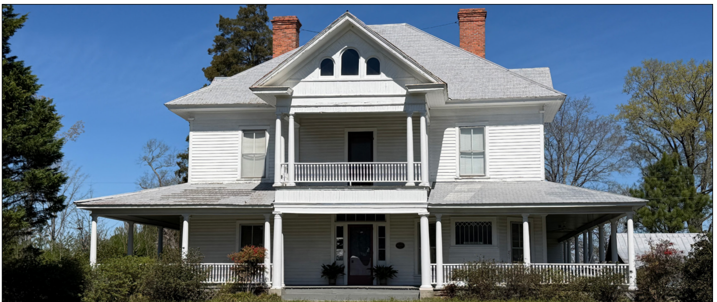
Routine maintenance forms the basis of responsible stewardship, protecting historic landmarks by addressing deterioration early and reducing the need for extensive repair or replacement. Samuel Bartley Holleman House near Holly Springs. Photograph by Capital Area Preservation, Inc.
