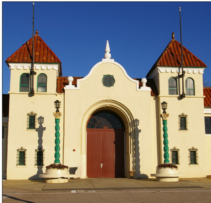
The North Carolina State Commercial and Agricultural Building features exterior stucco, a red clay tile roof, a masonry parapet, and other decorative masonry elements. Photograph by Capital Area Preservation, Inc.
