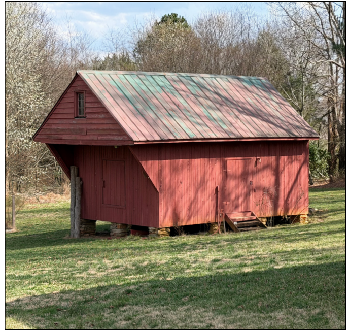
A small raised red barn on stone piers at the Thompson House near Wake Forest. Photograph by Capital Area Preservation, Inc.
