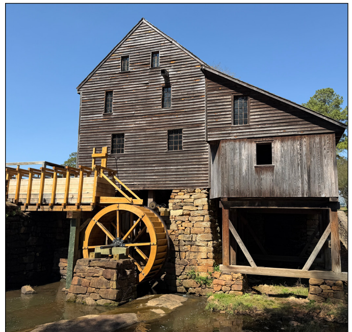
Yates Mill with its newly installed replacement waterwheel. Photograph by Capital Area Preservation, Inc.
