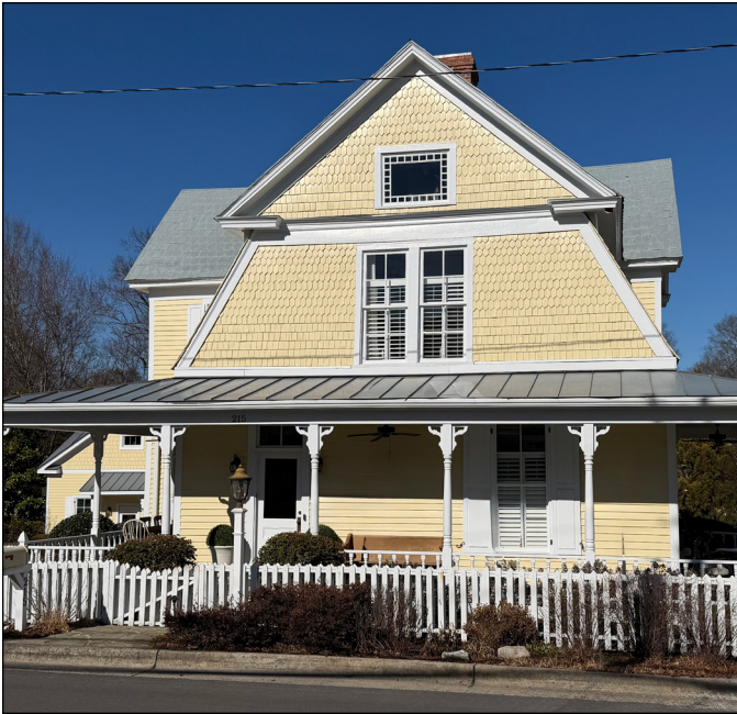
Contrasting trim accents the gambrel roof and facade detailing of the Harward House in Apex. Photograph by Capital Area Preservation, Inc.
