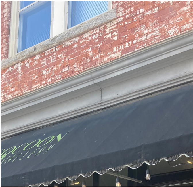
The metal cornice trim above the storefront window of the Hinton and Son Hardware Store in Apex is a character-defining architectural feature. Photograph by Loggia Preservation, 2025.
