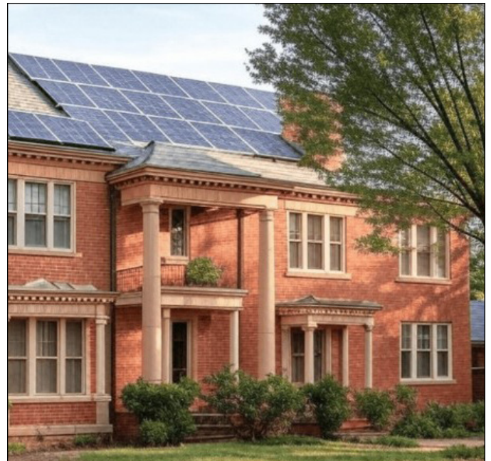
Solar panels must not be installed on primary facades, primary roof slopes, or highly visible elevations. Image from Google.
