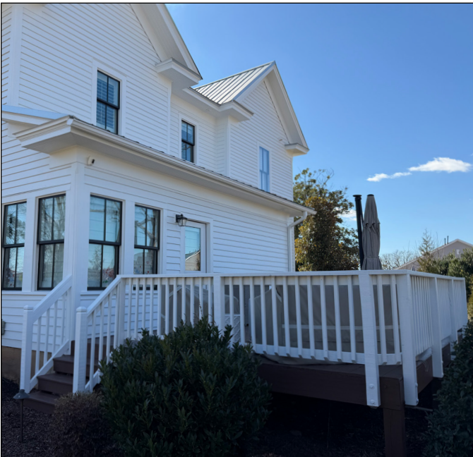
A simple deck on the rear of the Alsey Thomas Olive House in Apex minimizes the visual and physical impact on the landmark building. Photograph by Capital Area Preservation, Inc.
